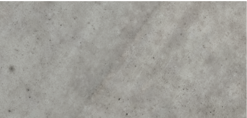
FLOAT FINISHED CONCRETE
